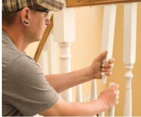
\*\* Note – If your old wooden balusters did not use nails, but used a Dowel Pin and Wood Glue, there is a possibility that you could break off part of the tread / floor and/or handrail along with the baluster. Some installers will cut the wood balusters off at the top and bottom and then sand it smooth. Others will replace the handrail and tread if irreparable damage has occurred.
